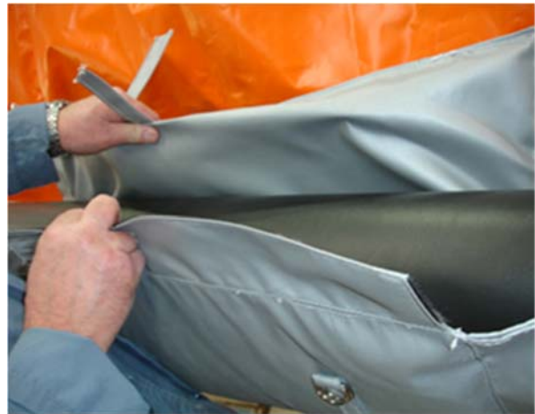
Release and wrap circumferentially around the pipe
