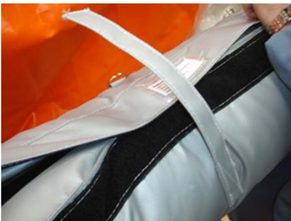
Catch the Velcro at various points along the length to temporary hold in place
