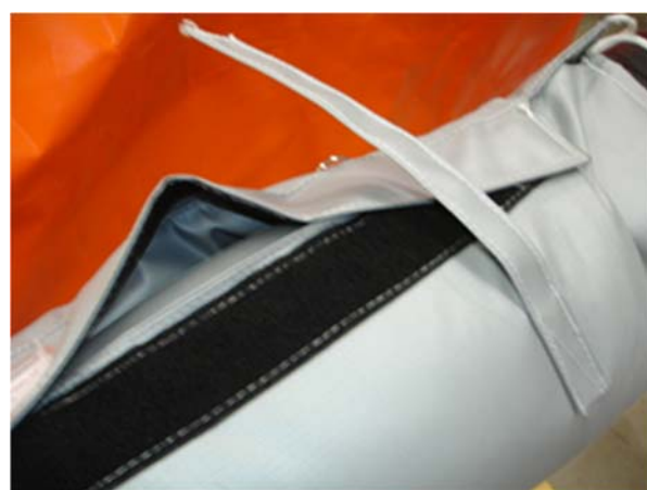
Catch the Velcro at various points along the length to temporary hold in place
