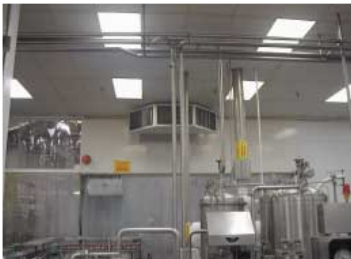
The carbon dioxide exhaust fans in the filler room are capable of 15 air changes per hour at Springs Inc., which is a major soft drink manufacturer and a large local Coca-Cola franchise distributor located in Huntsville, Alabama.
