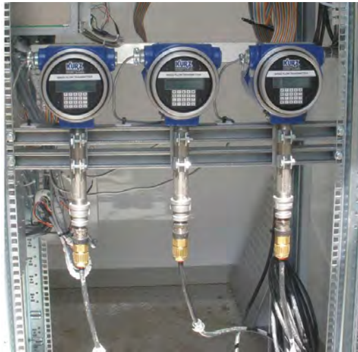
Figure 2-21. Cable gland example with braided shielded cable
