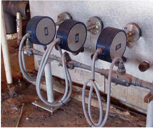
Figure 2-19. Flex sensor connection for service loop, TA version using liquid tight conduit
