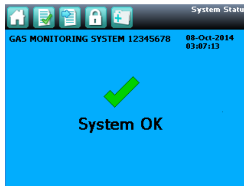
Figure 30. System Status Normal
