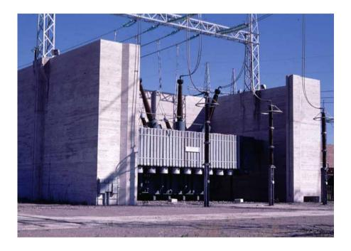
Transformer windings are insulated with cellulose and surrounded by oil to ensure proper insulation and cooling. Poor oil quality can lead to a low dielectric strength and even to a system failure. High water content together with dissolved gases in oil may cause bubbling in case the total pressure of gases exceeds the ambient pressure of the transformer.
